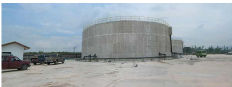
Figure 7. Biogas digesters in a cassava factory developed by KMUTT.
