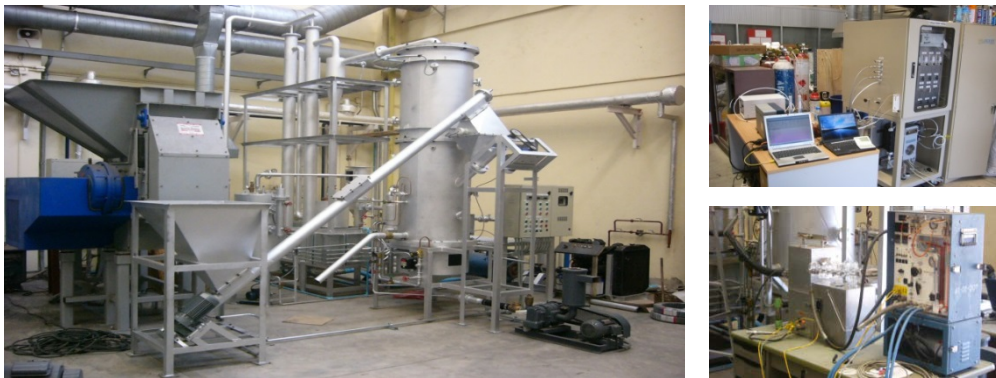
Figure 5. Bubbling fluidised bed gasification facility at JGSEE.
